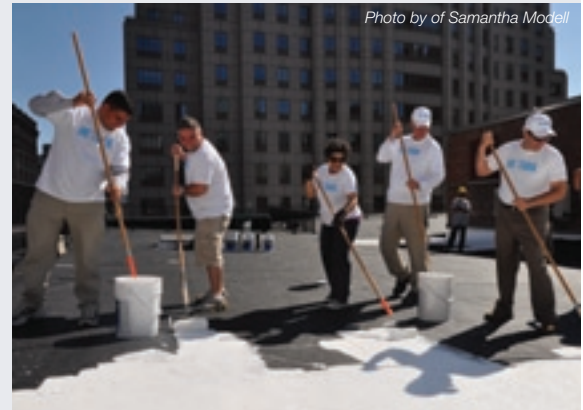
Volunteers participating in the NYC °Cool Roofs Program paint an urban rooftop with a cool roof coating.
