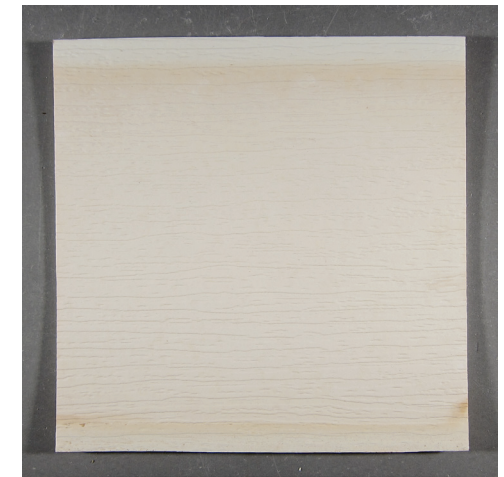
Yellowing of a white vinyl siding material
