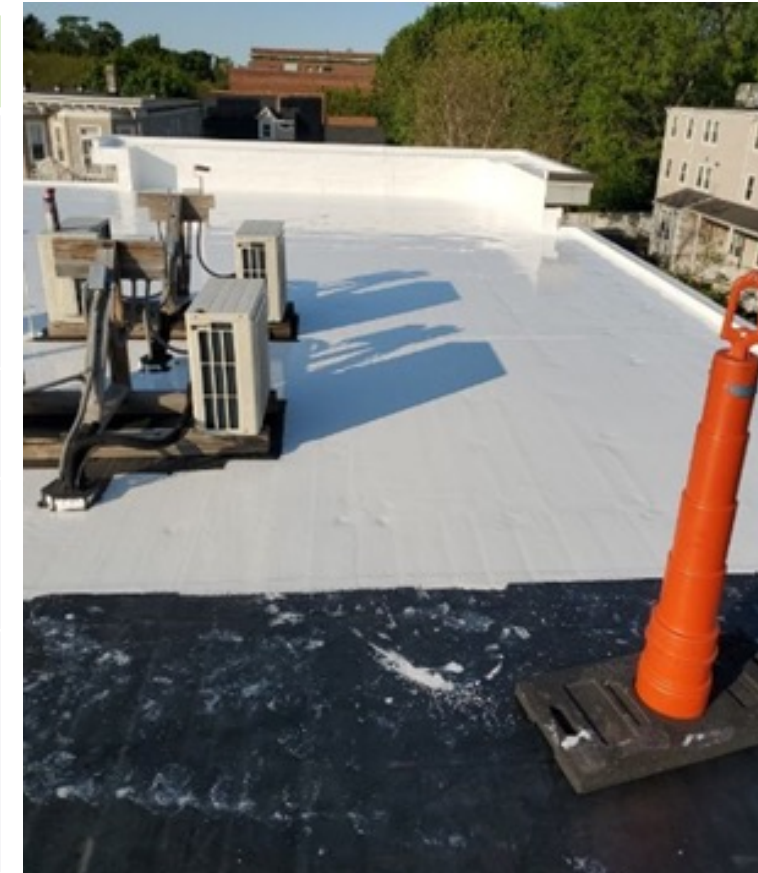
Pine Street Inn Reflective Coating Installation
