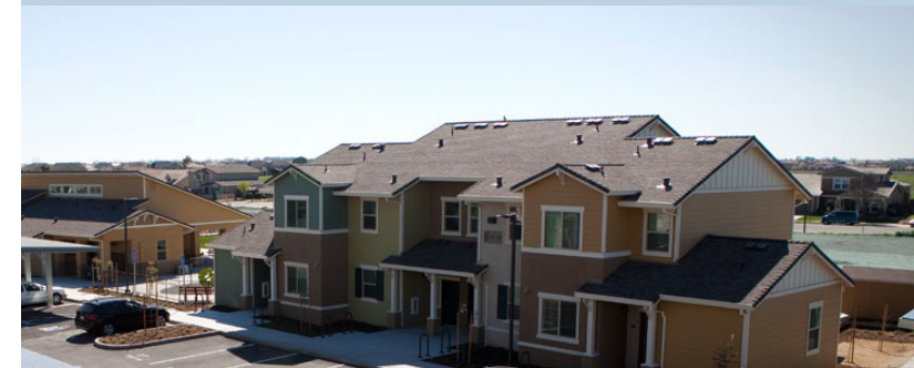
Asphalt shingle cool roof at Mutual Housing at Spring Lake.
