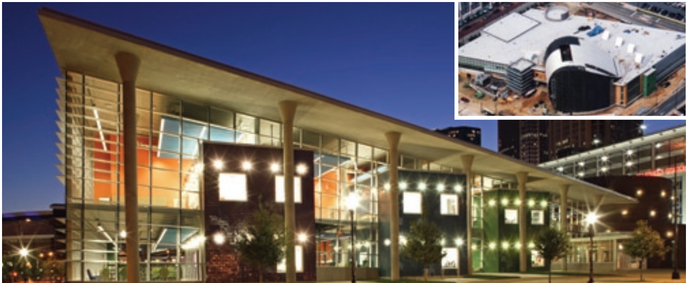
A cool roof slopes from one end of ImaginOn: The Joe & Joan Martin Center in North Carolina to the other. Construction photo in the inset shows the many ways this roofing system was installed to accommodate skylights, slopes and a flat roof surface. This project received a LEED-NC Silver rating in 2006 receiving the LEED 7.2 credit for the mitigation of heat island effects. [Photos courtesy of Gantt Huberman Architects, PLLC. Photography (left) by Tom Kessler Photography.]
