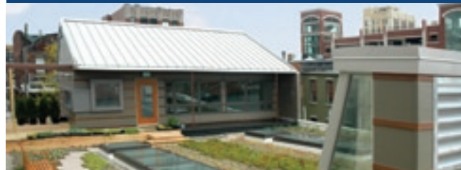
A green retreat allowed the architect to test various types of cool roofs and sustainable design strategies, including this sloped metal cool roof over the conference room. (Photo courtesy of A3C Collaborative Architecture.)
